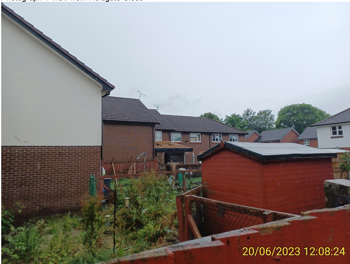
Photograph 2 View from Holdgate Close car park area
